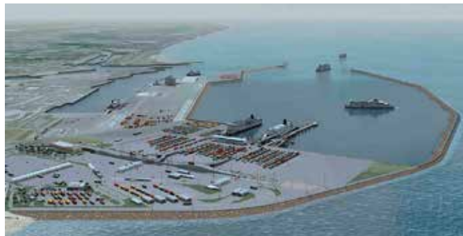
Artist's rendering of the new coal port at Nacala, Mozambique, from consultant Arcadis, which is advising on the scheme. (Image: Arcadis)
