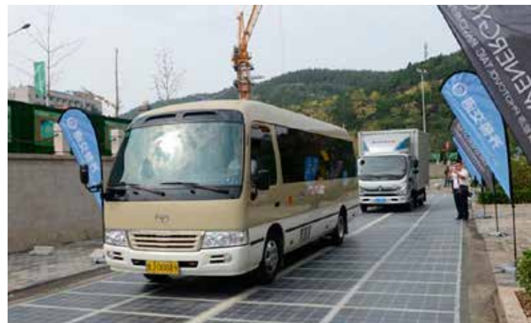
Jinan City's solar roadway will be durable enough to carry medium-sized trucks.
