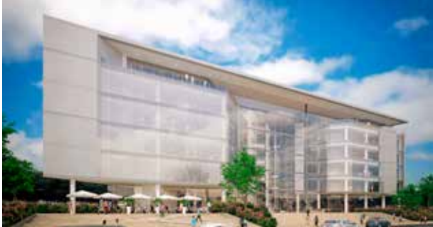
Concor Buildings has secured the contract for the construction of Phase 1 of Oxford Parks.
