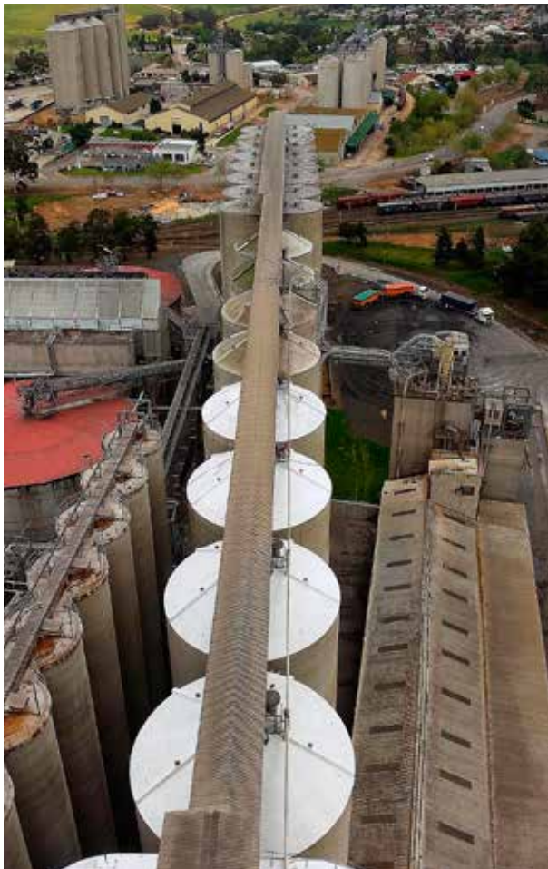
Inspection of the Caledon breweries' silo roofs and work in progress on the refurbishment project for which a.b.e. Construction Chemicals supplied a variety of products.
