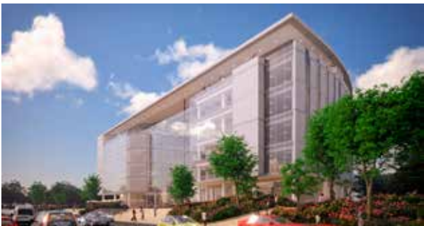
Being developed by premier property development company Intaprop, Oxford Parks is set to become a vibrant mixed-use precinct.
