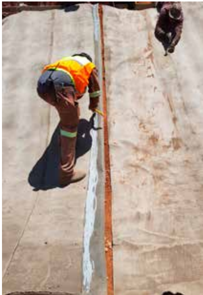
Applying the transparent hybrid adhesive on Concrete Canvas overlaps.
