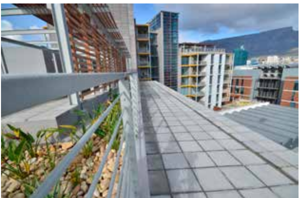
Revelstone's Jura paver was used extensively on the eighth and 12th floor sundecks. (Photo by David Beer)
