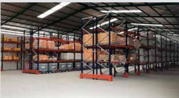
Warehouse of Sika's new plant in Cameroon.
