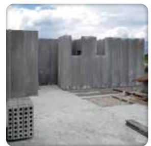
Erected Partition Wall Panels
