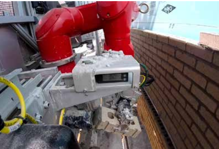
A bricklaying robot in action.
