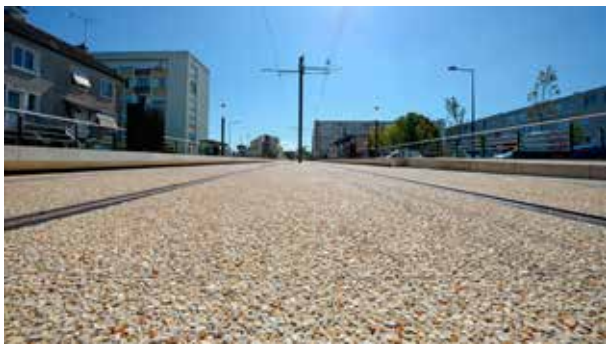
Protective products applied to concrete will protect against traffic, greasy stains, micro-organisms and UV rays.
