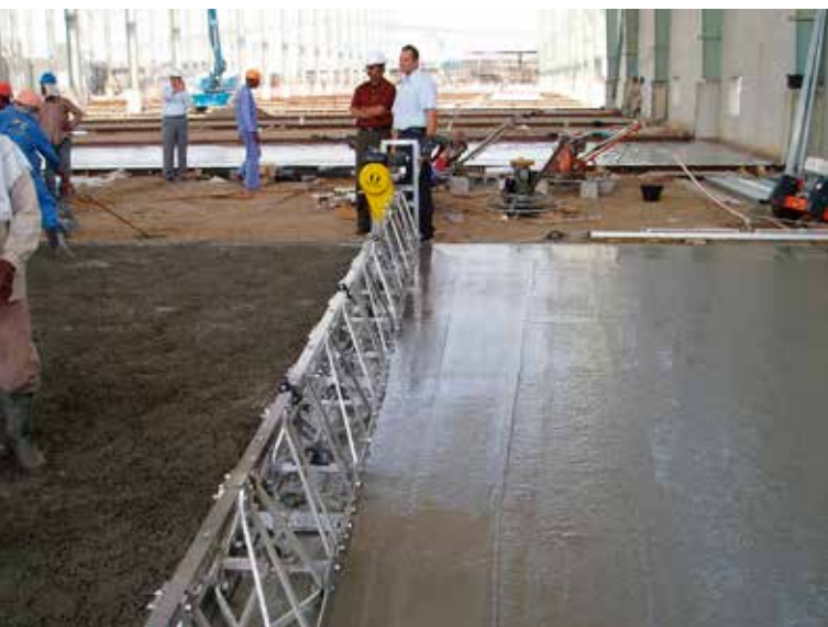
Levelling and compacting with a vibrating truss.
