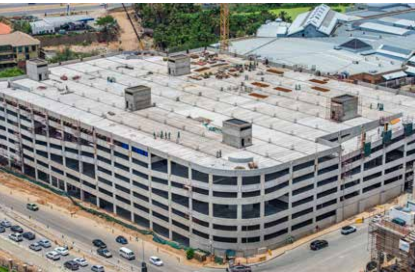
An aerial view of the parkade under construction.
