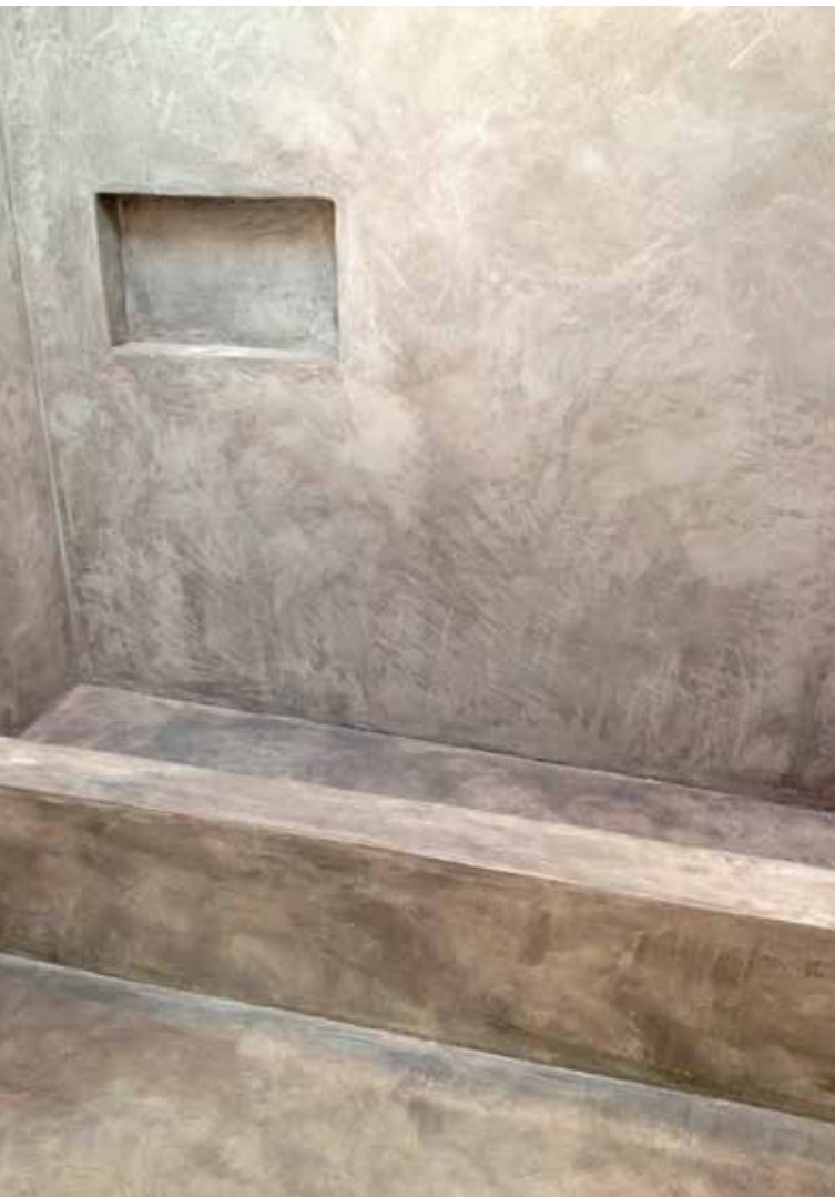
a.b.e. Construction Chemicals' duraproof cem block is a powdered cementitious waterproofing product that is easy to use and streamlines the waterproofing of plaster and mortar.
