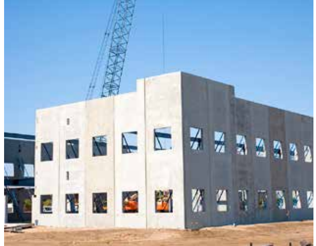
A stack-cast structure with panels being lifted by crane.
