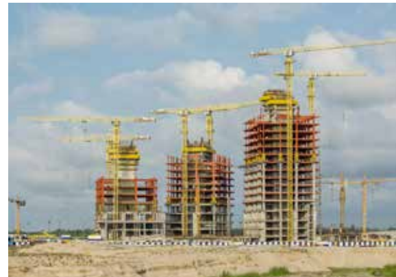
58 Construction of Azuri Peninsula, Nigeria.
