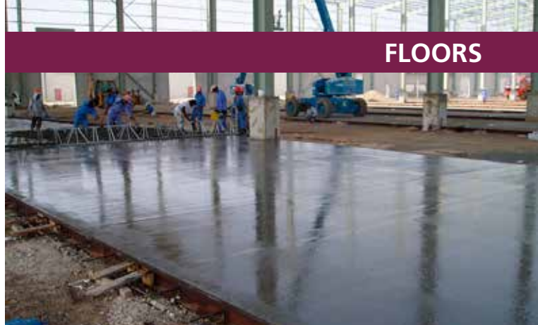
Compacted concrete awaiting finishing.
