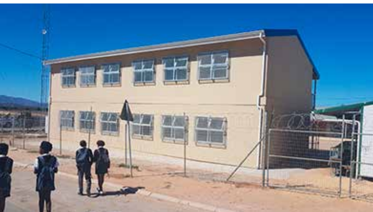
A double-storey classroom built for the Western Cape Department of Education.
