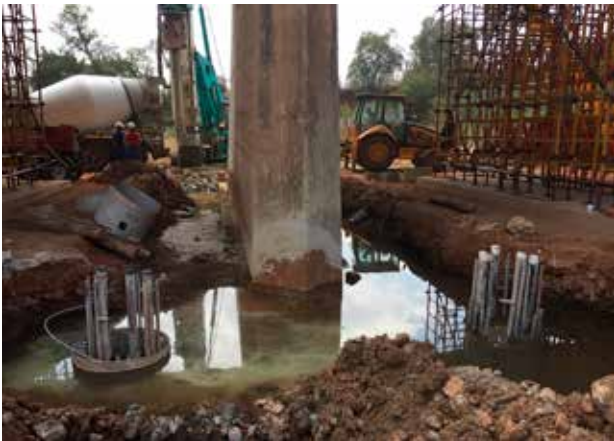
Installation of the piles.
