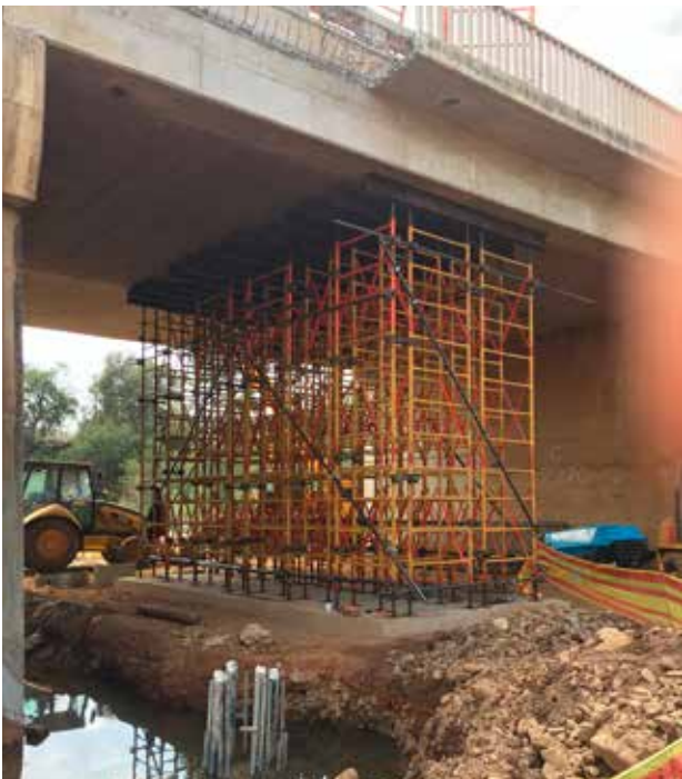
Excavation for the construction of the concrete beam.
