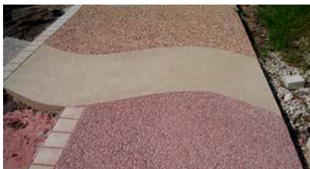
Exposed aggregate concrete gives a warm and natural look.
