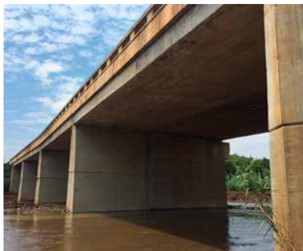
The repaired pier and reinstated riverbed.
