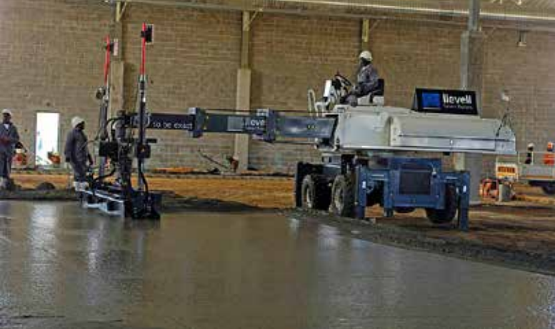
Levelling and compacting with a laser screed.
