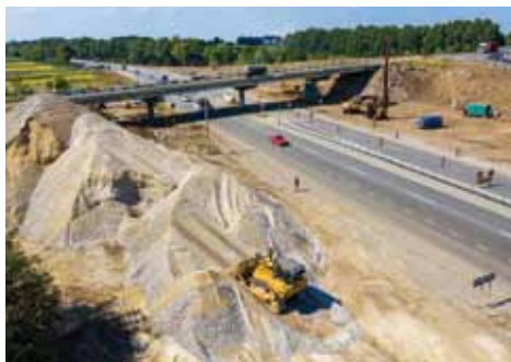
For pump concrete one needs filler sand and an admixture can compensate for the lack of sand to give it flow.
