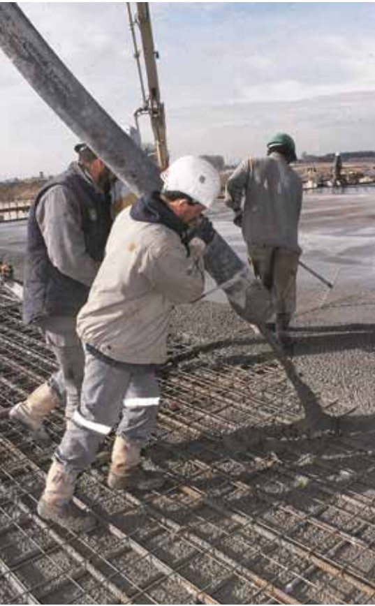
Admixtures improve concrete quality, manageability and acceleration or retardation of setting time.
