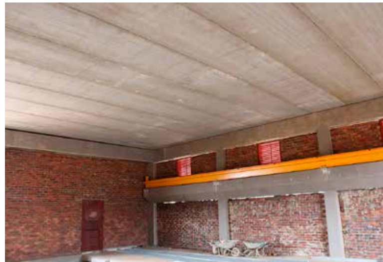
The high-quality hollow-core slabs were manufactured using state-of-the-art extrusion technologies at the company's precast concrete factory.
