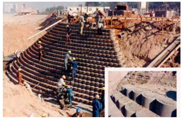
CRB beach protection at Laguna beach near the Umgeni river mouth.
