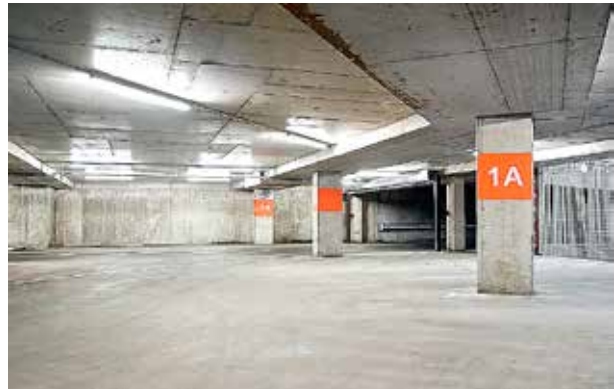
A heavy-duty parking-garage floor.
