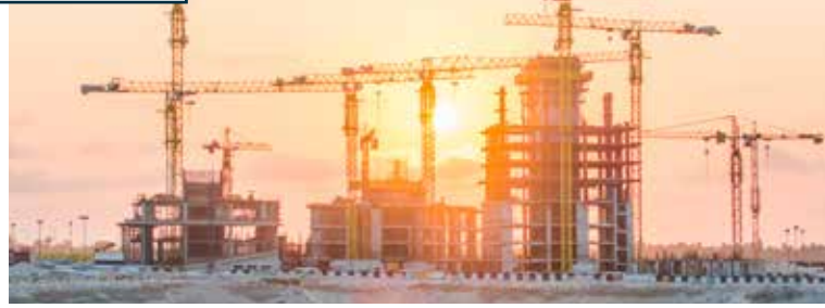
The cranes are working 24 hours a day.
