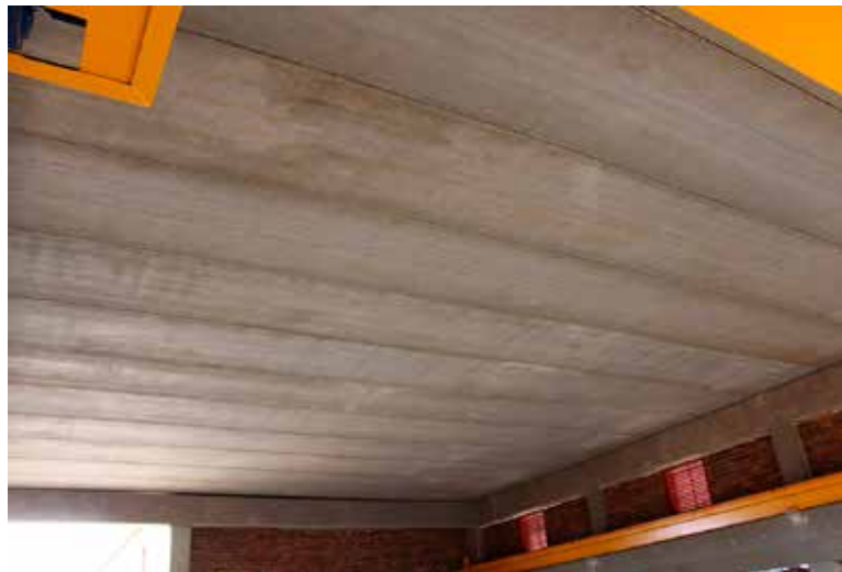
The high-quality hollow-core slabs were manufactured using state-of-the-art extrusion technologies at the company's precast concrete factory.
