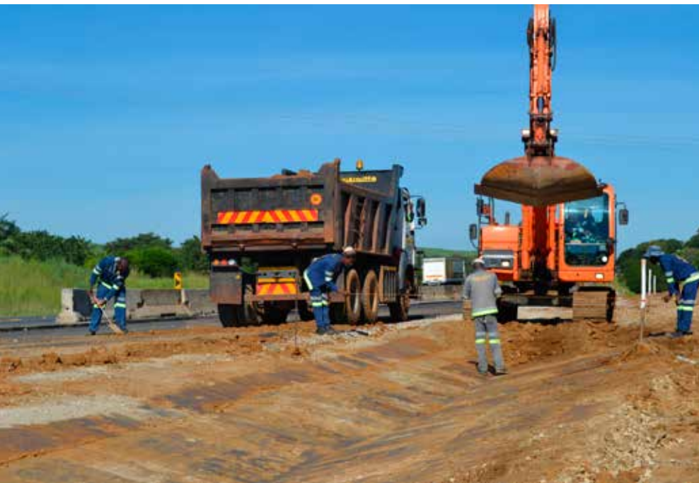
Construction of side drains in progress.
