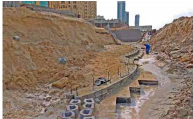
Beach front protection with Terraforce, Fairmont Hotel, Ajman.
