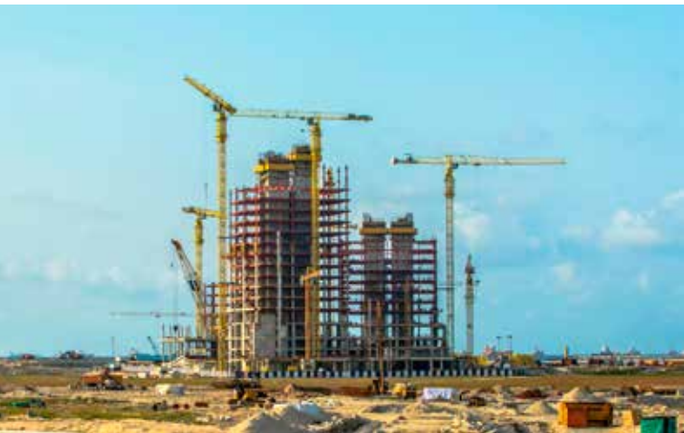
The cranes at Azuri Peninsula were equipped with the Effi-Plus system which increases hoisting speeds with light loads and below the COMANSA cranes are now working at their maximum height, the tallest reaching up to 163.5 metres.
