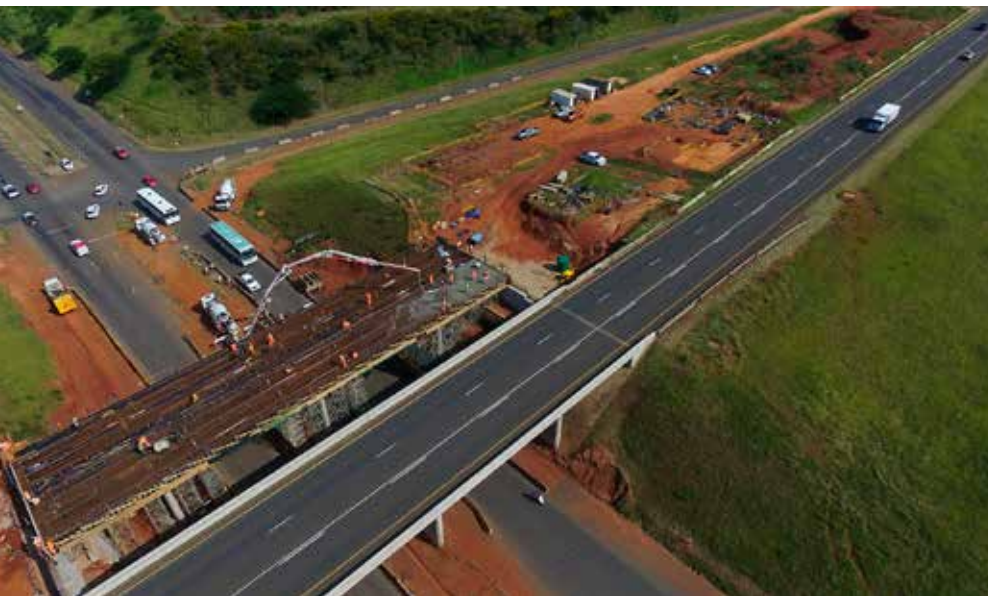
Concrete pour in progress on the Empangeni T-junction overpass deck.
