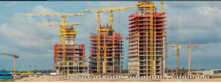
All 6 COMANSA cranes have flat-top design and maximum load capacity of 18 and 20 tonnes.
