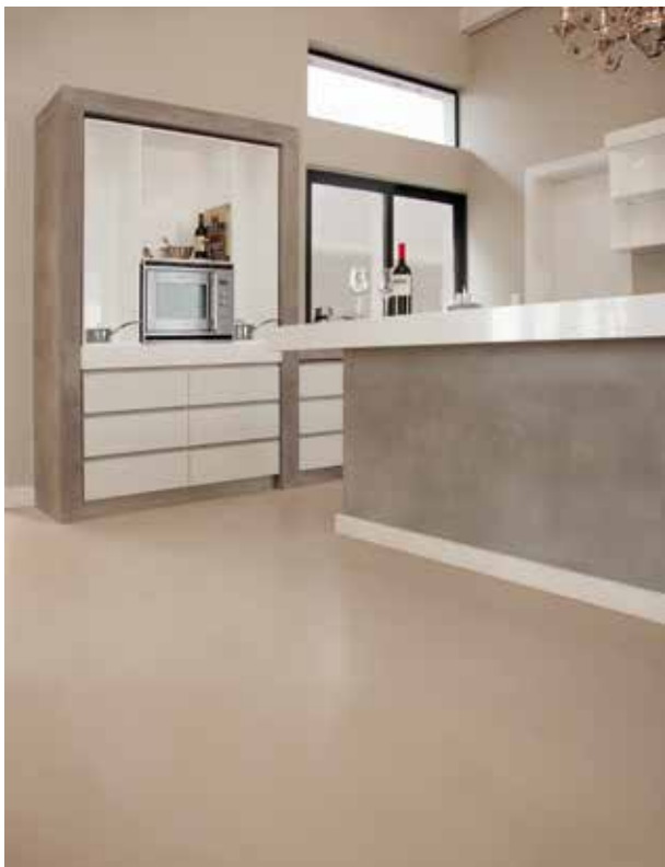
For a smooth floor surface with a homogenous finish in a range of colours TAL SuperFlow decorative overlayment is ideal.
