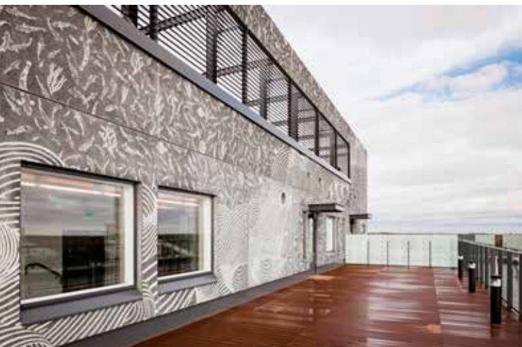
Residential building Espoon Tähystäjä in Espoo, Finland, has a decorative concrete façade – an artwork of underwater creatures and giant waves by Finnish artist Aimo Katjamäki. Photo: Graphic Concrete.
