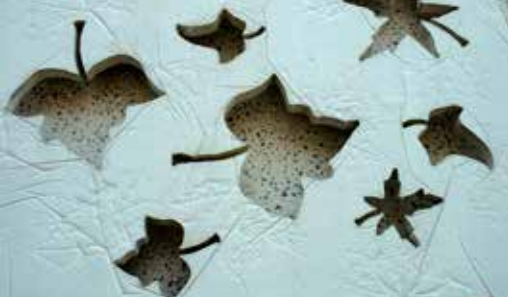
Premoulding oils, if used when casting concrete, will raise the quality of finishes and extend the life of formwork
