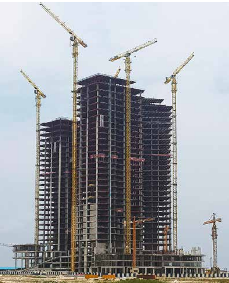
The cranes at Azuri Peninsula were equipped with the Effi-Plus system which increases hoisting speeds with light loads and below the COMANSA cranes are now working at their maximum height, the tallest reaching up to 163.5 metres.
