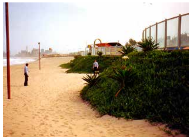
The 6-m-high wall has been very effective in protecting the pools installed immediately behind it.
