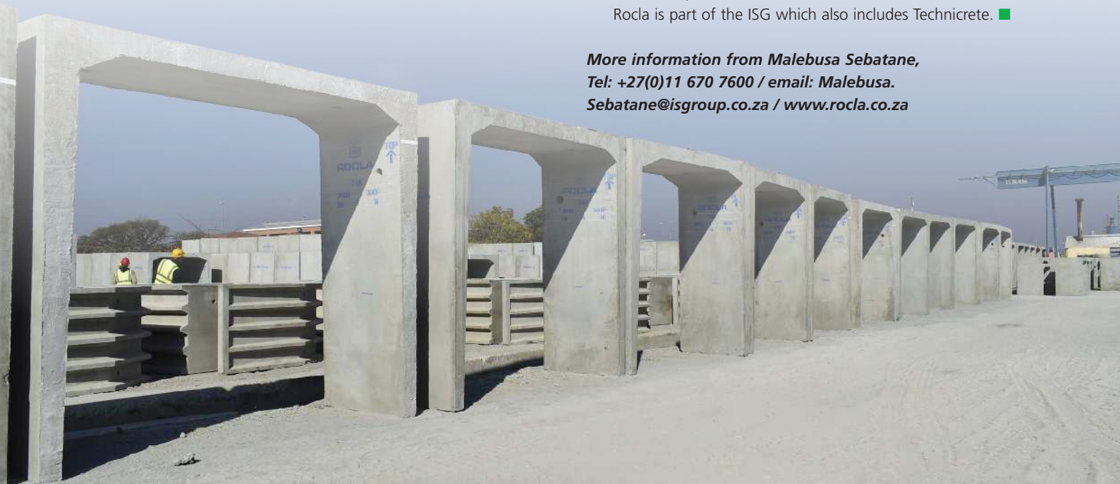
Culverts are integral to water, road and mining infrastructure.
