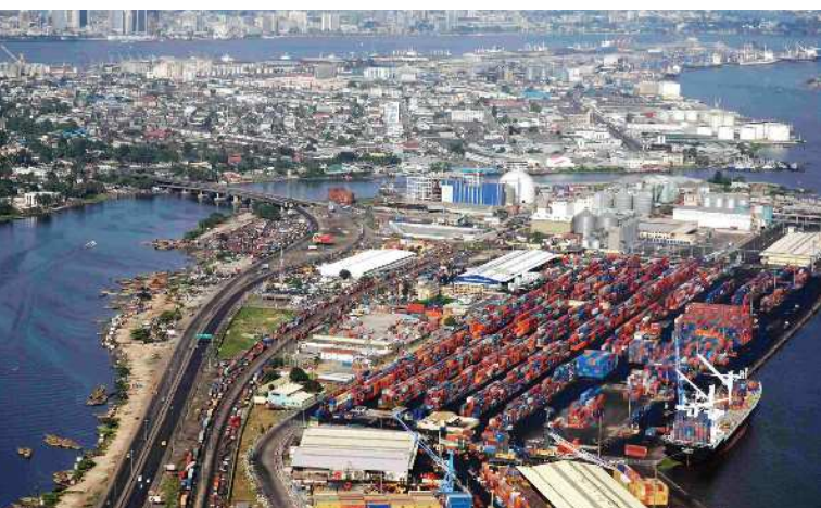
Port of Lagos, Apapa – the largest container terminal in Nigeria (Global Construction Review, 2017)
