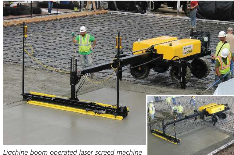
Ligchine boom operated laser screed machine
