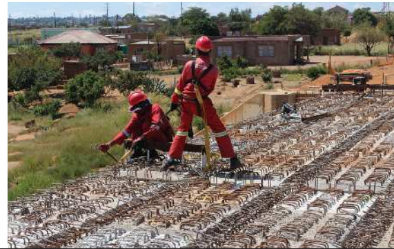
14 Constructing a bridge over the Mankgatle River
