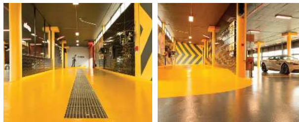
The Machine WashWorx floors convey the company image while meeting challenging cleaning activities.
