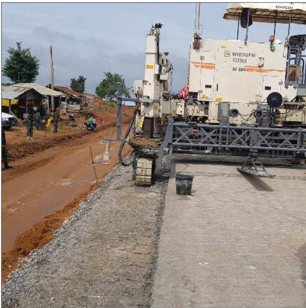
The construction arm of the Dangote Group is laying durable concrete roads in Nigeria.
