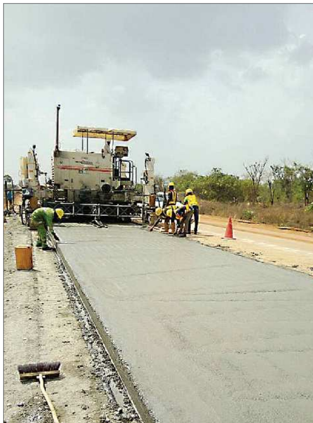
Africa is starting to accept concrete roads for their long-term minimum-maintenance durability.
