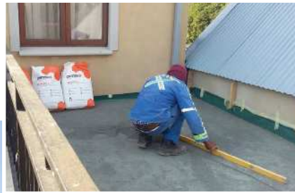
ScreedLite being placed on a roof deck as a lightweight screed.
