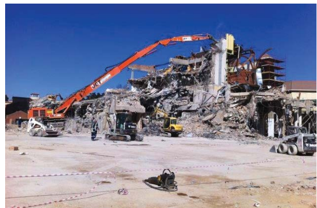
Demolition provides a continuous challenge in terms of safety
