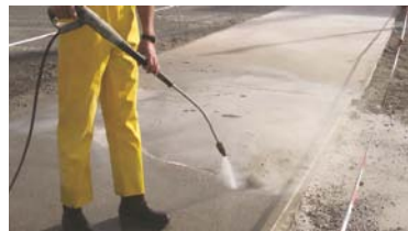
Applying a curing compound from the CHRYSO® Cure Range to the precast segments reduces the incidence of shrinkage cracks
