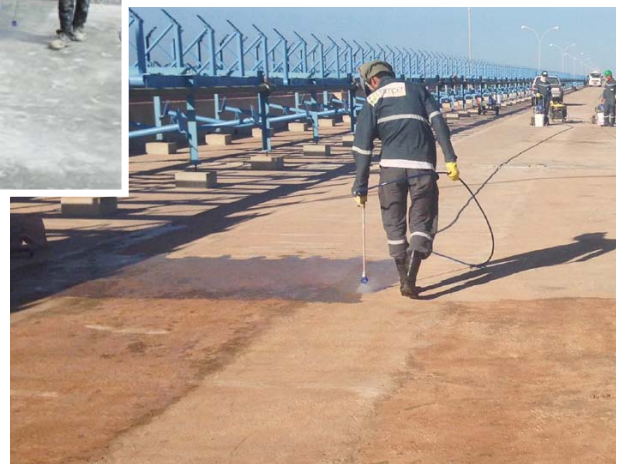
SCP can enhance the life expectancy of concrete by as much as two to three times
