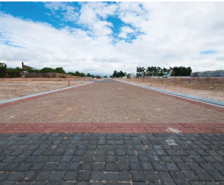
Inca Concrete Products’ Tan Exposed Aggregate interlocking pavers and its Twin-block Cobble are used creatively on Bonsai Estate’s roads
