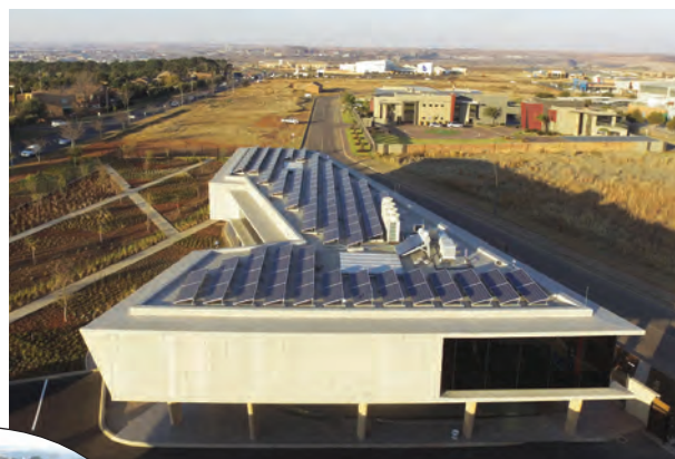
▲ View over the GLPS building looking East showing PV cells and roof services. Photographer: Frederik Botha
