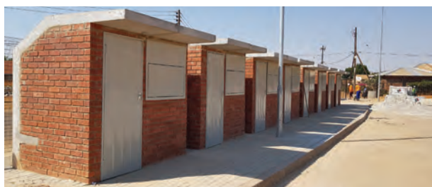
Some of the Rocla precast concrete bus shelters were converted into hawkker stalls.
