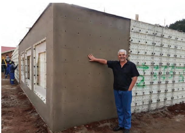
Hennie Botes inventor of the moladi plastic formwork.
