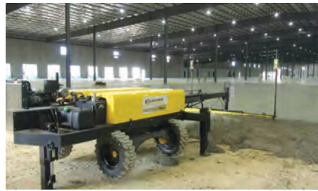
The Ligchine boom operated laser screed machine
