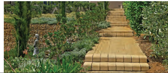
24 Retaining walls at Hidden Valley Wines
