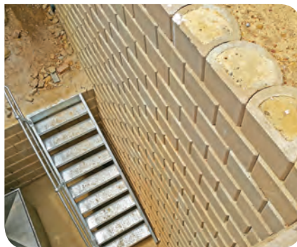
The fat trap constructed for the Overture restaurant.
