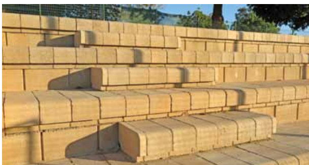
Some steps capped with the Terraforce Four x Four® Step Block Caps.
