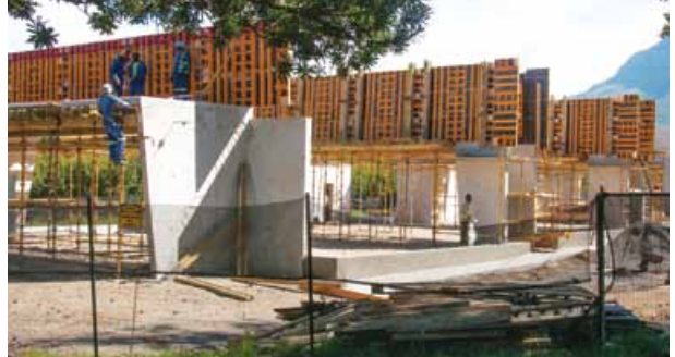
Shuttering for the in-situ roof slabs straddles the U-shaped precast concrete elements.
