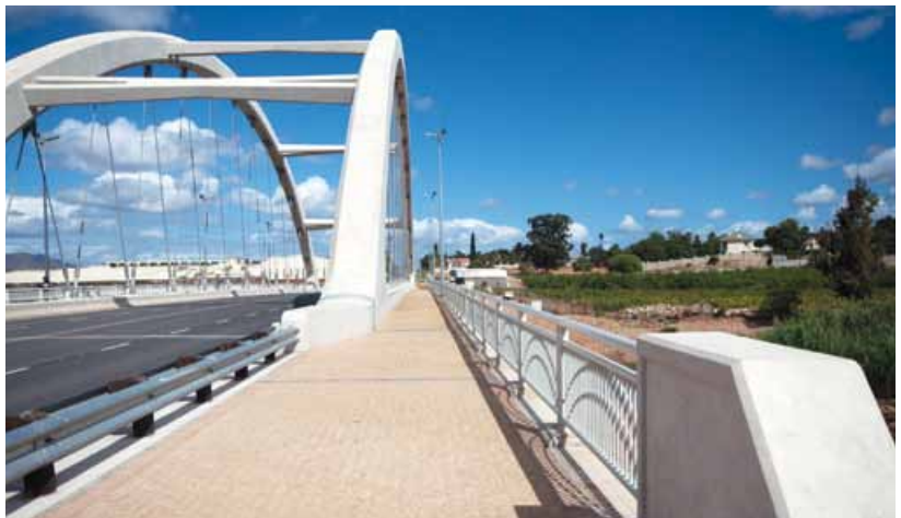
A sidewalk paved with C.E.L.'s coarse-exposed aggregate pavers on Ashton's recently completed cable-tied-arch bridge.
