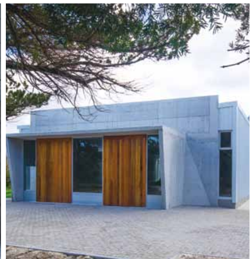
The southern barn-door car entrance mounted between two of the precast concrete elements supplied by Cape Concrete.
