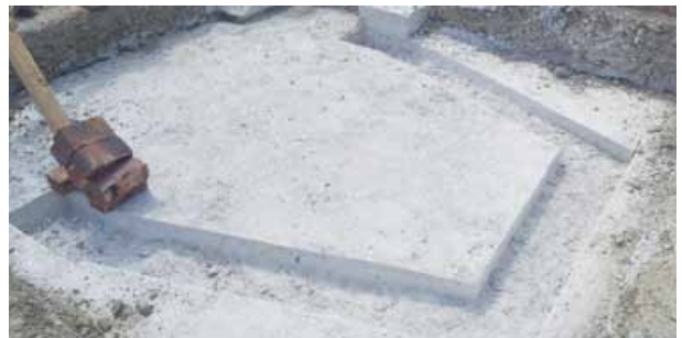
One of the U-shaped footing channels.
