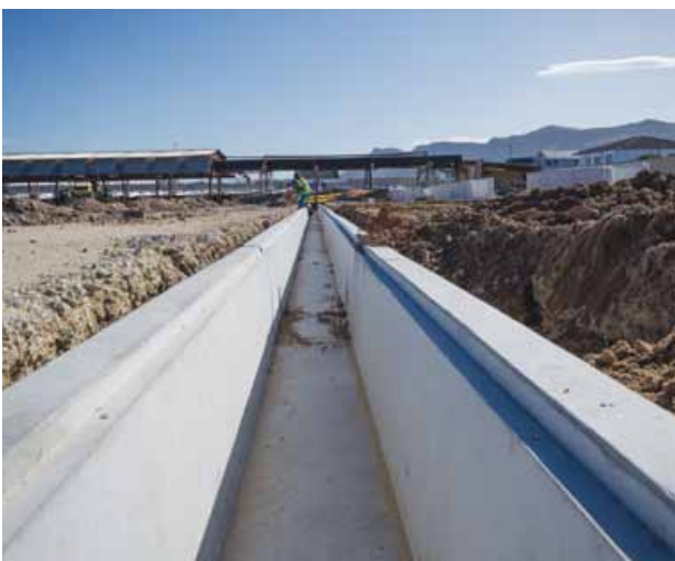
Freshly laid precast concrete channels.
