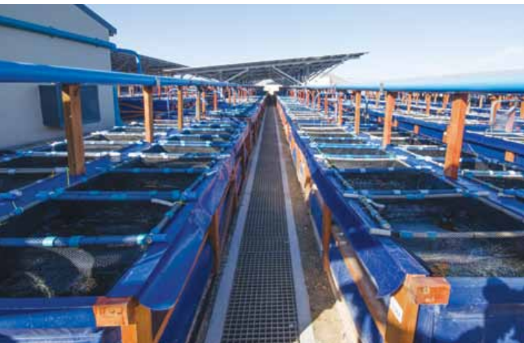
A precast concrete drainage channel flanked by two rows of abalone tanks.
