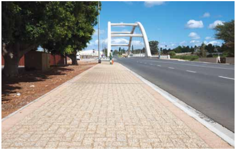
A sidewalk in Ashton paved with C.E.L.'s coarse-exposed aggregate pavers.
