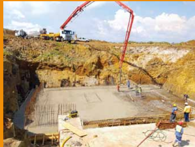
Foxcrete 37m Kusha foundation
