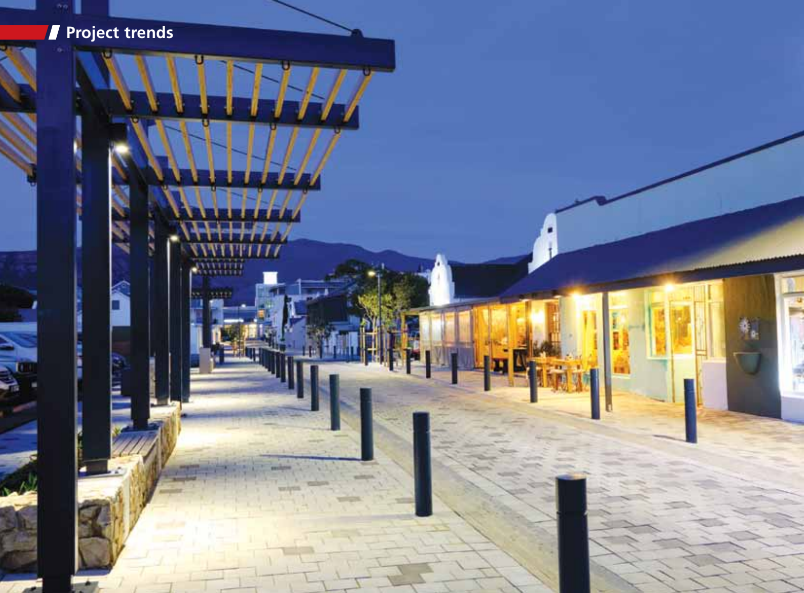
Some of the paving layouts and newly planted trees.
