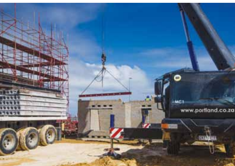
One of the steel beams being offloaded.
