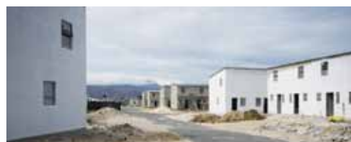
Partially completed double-storey houses at Lourensa Park.
