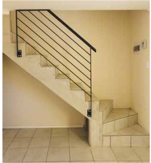
A fully completed precast concrete staircase.
