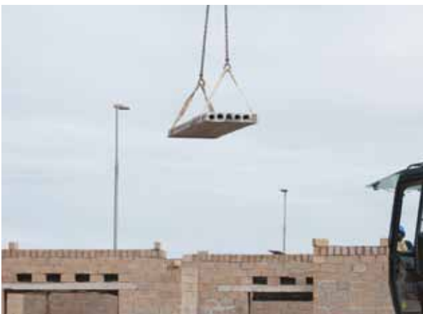
A hollow-core slab is lowered into position.
