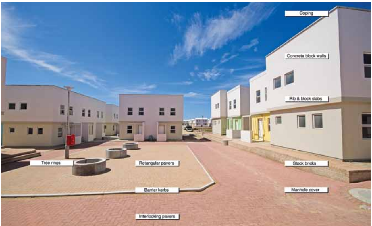
Apart from its precast staircases, this picture shows the entire range of products delivered by Mobicast to Mountain View.
