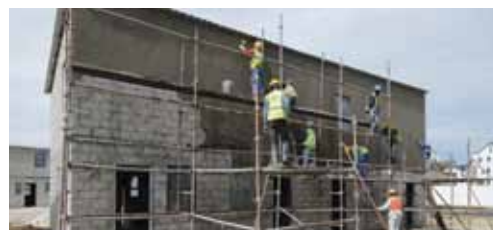
A double-storey unit under construction.
