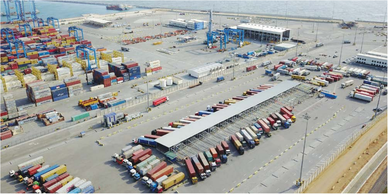
AECOM is on track to complete its scope of work at Tema Port in September
