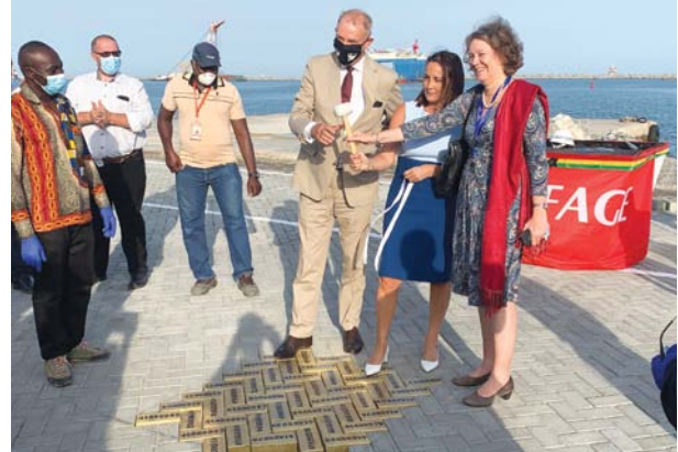
An official ceremony to mark the completion of the heavy duty paving
