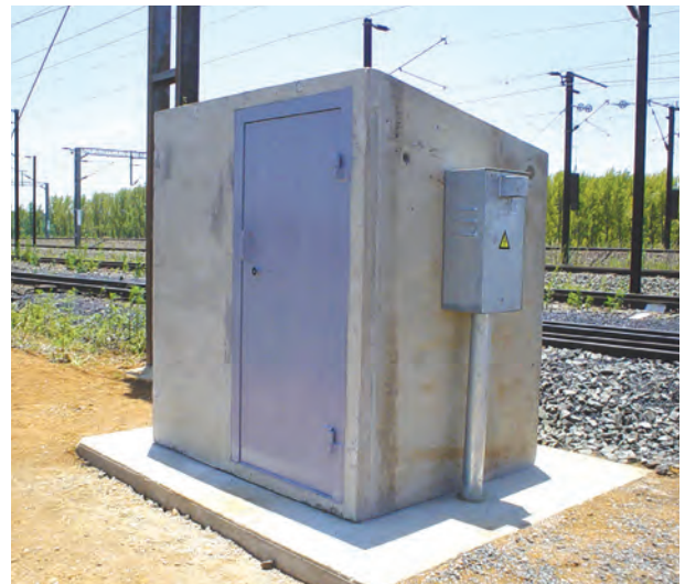
Security box shelter.
