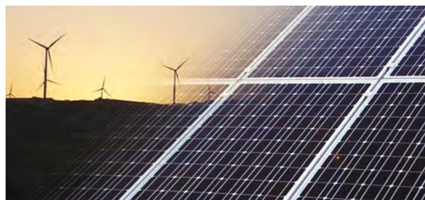
Hybrid renewable power plant
