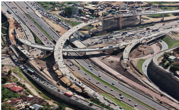
The award-winning Umgeni Road interchange.
