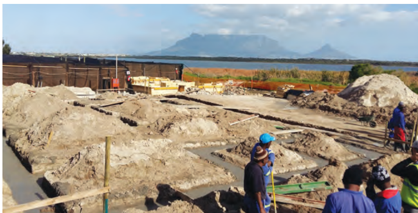
Foundation to start building penguin pools.
