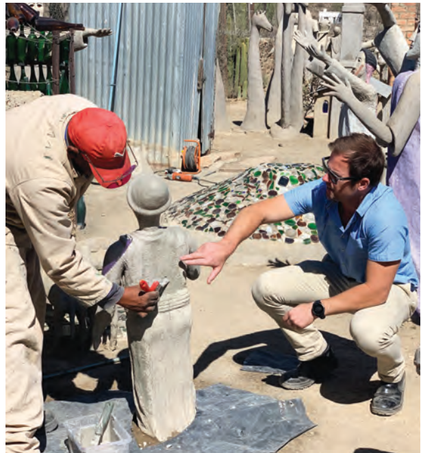
Renovation work to sculptures was made possible by using advanced concrete rehabilitation products generously supplied by Chryso and a.b.e.
