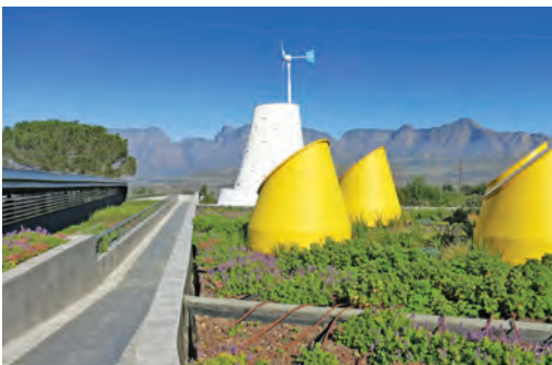
Roof garden, skylights and wind turbine.
