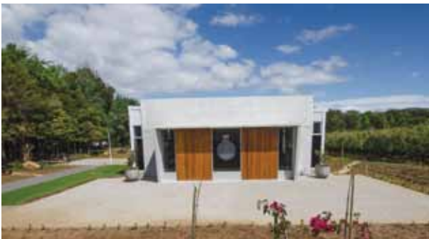
The north-facing vehicle entrance.
