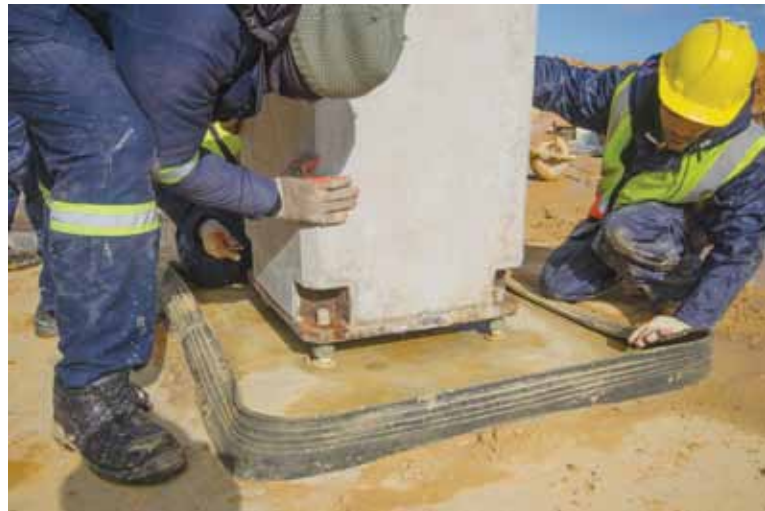
A precast column is lowered onto the connecting bolts.
