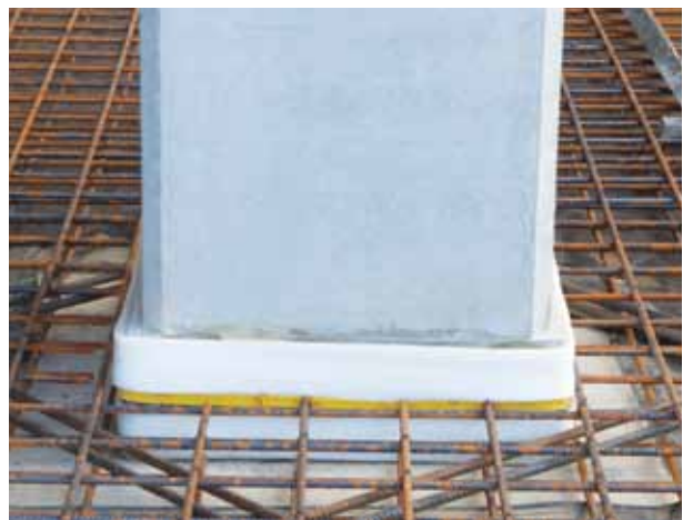
A grouted column base showing the yellow Sikaswell Water-Stop.
