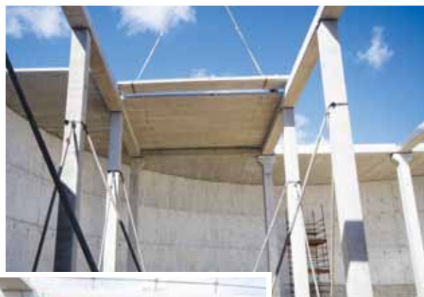
▲ A hollow-core slab is lowered into position.
