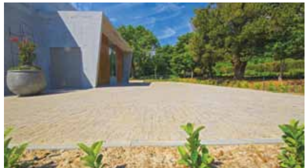
The paved driveway and vehicle entrance at the southern end of the museum.
