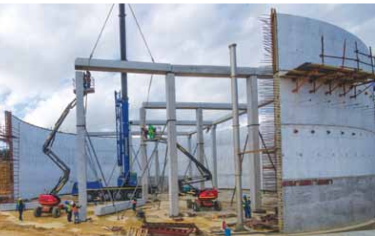
A precast beam is lowered into position.
