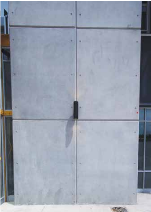
The panelling shortly after installation.
