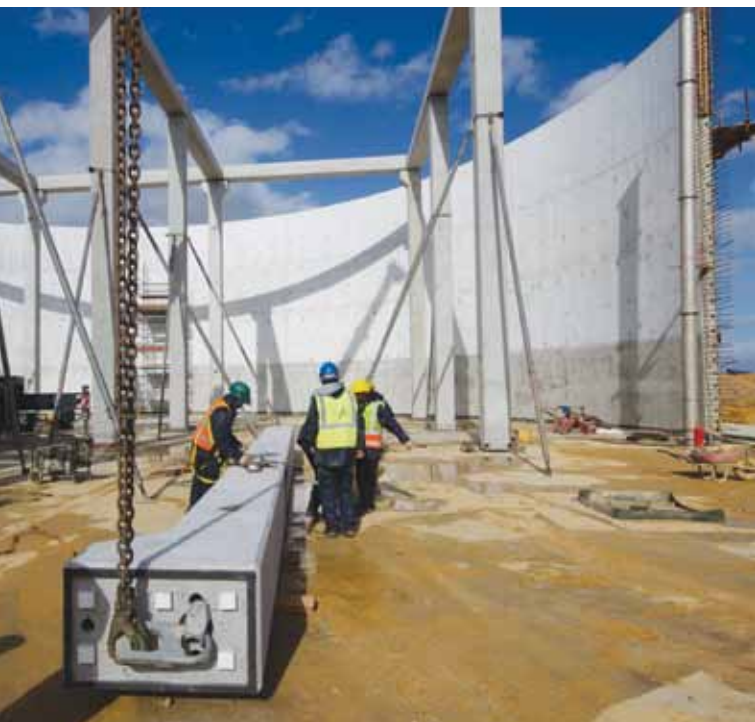
A precast column is prepared for lifting into position.
