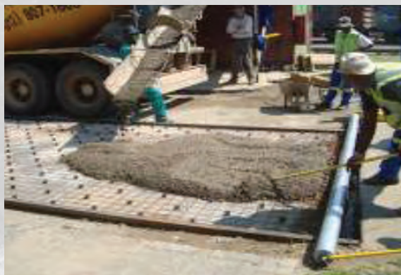
Casting of concrete
