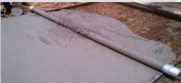
Spreading of concrete with spin roller
