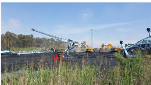
Demolition of redundant mining infrastructure
