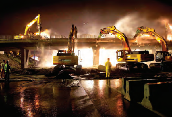
Overnight bridge demolition over a highway
