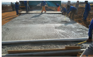
Spin roller level out wet concrete
