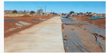
Curing the UTRC under plastic sheeting
