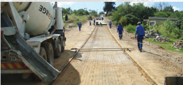
Mesh installed on spacer blocks, ready for concrete
