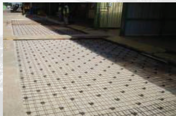
Preparation of reinforcing
