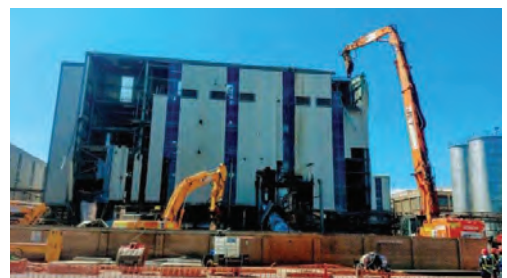
Flame-free high-reach demolition within a flammable environment
