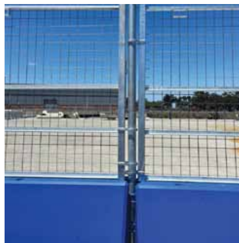
The pre-assembly of some barriers and fencing in Cape Concrete's yard.
