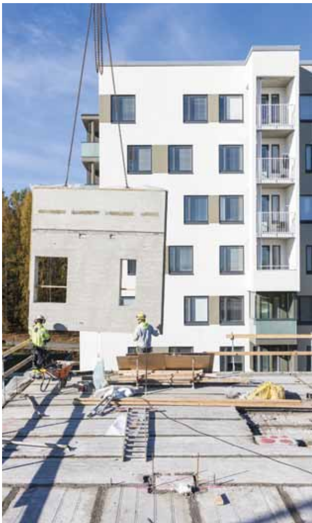
Building construction using precast flooring and walling.
