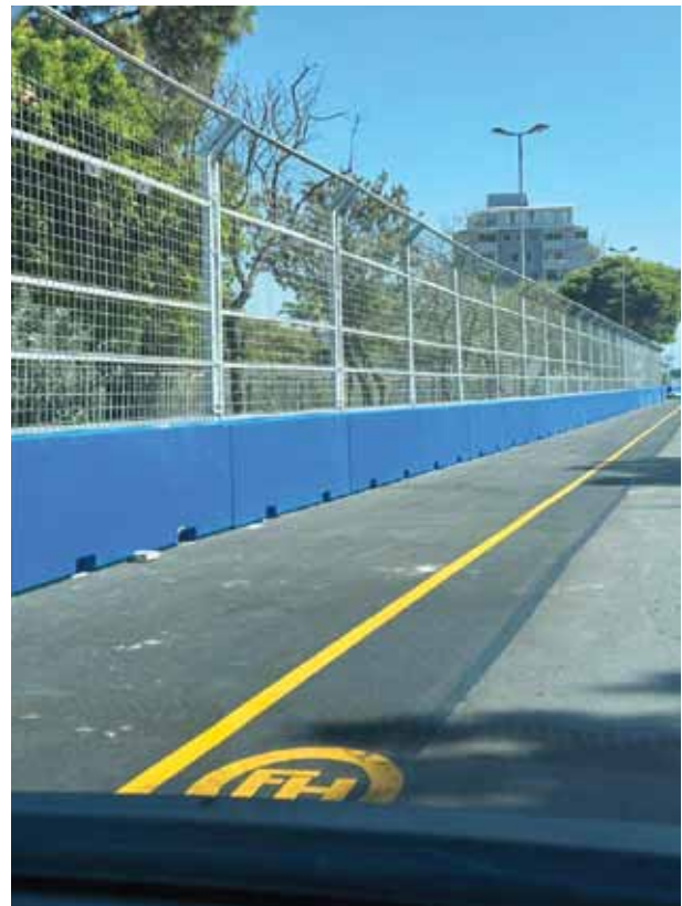
A barrier section on the Cape Town track.
