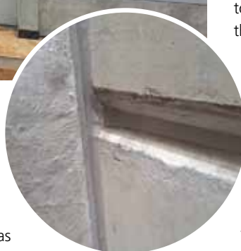
A section of the wall nears completion.
