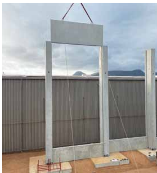
Precast concrete panels are lowered into position in the open area.
