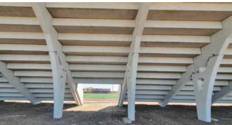
The grandstand was erected in as little as four months.
