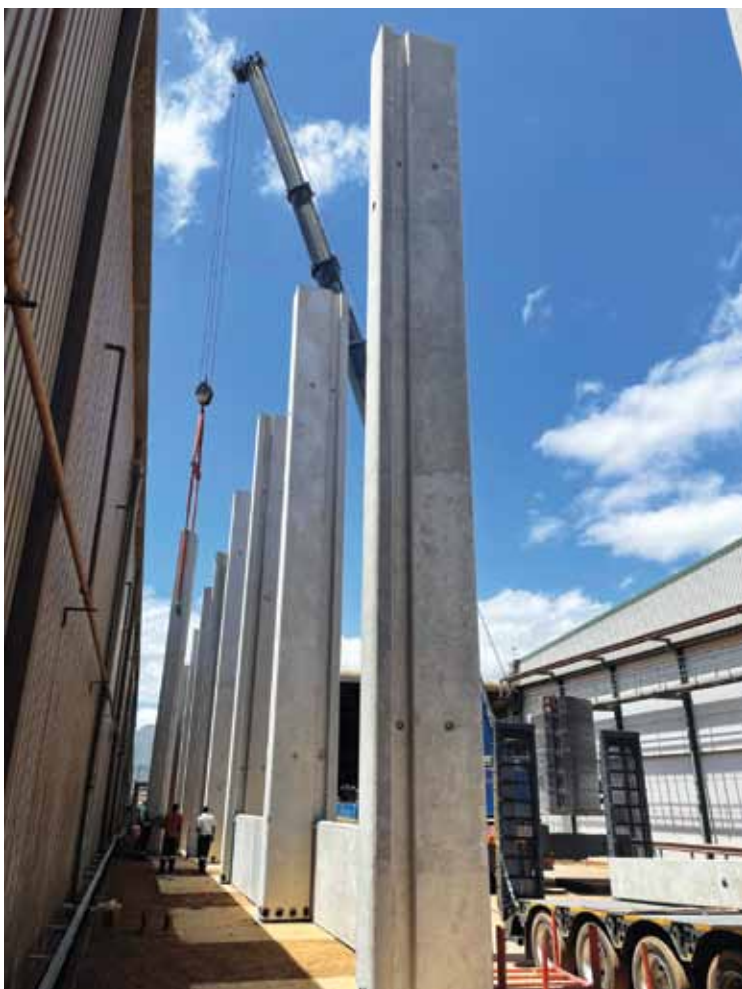
Precast concrete columns being lowered into position.
