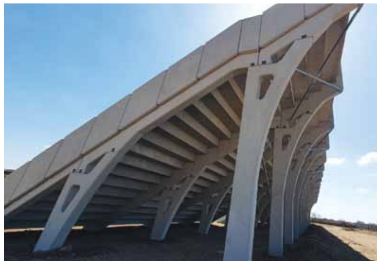
Constructing the grandstand in this manner has provided an almost 40% reduction in construction costs for the municipality.
